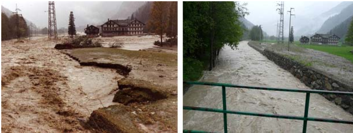
Dresal plain during the flood of 2000 (left) and during the flood in 2008, after the construction of protection measures (right) (photo RAVA).
